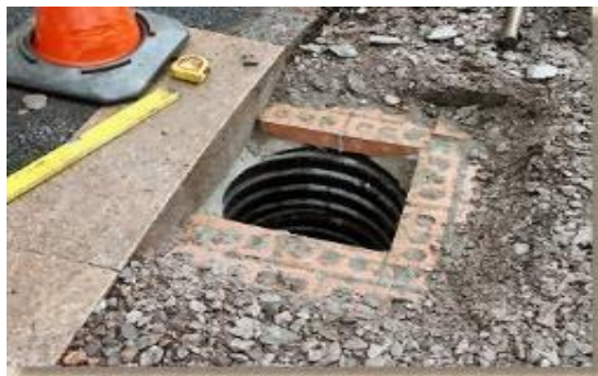
fig 6.Gully pot attached to underground drainage
