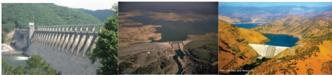
Fig. 1: A view of the CGD selected for modelling: the Bluestone Dam (Left); the Folsom Dam (Middle); Pine Flat Dam (Right) [15].
