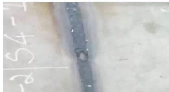
Fig.8 Automated Weld Joint
